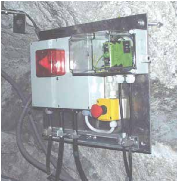
Fig.: Compact flashing light used for a safety application in a tunnel. The input voltage range of 70–264 V AC and 73–140 V DC supports both line (mains) and backup battery power
