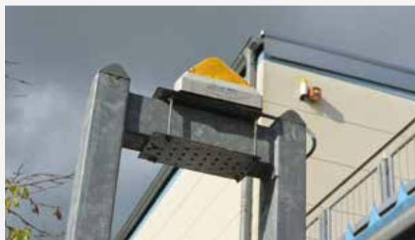
Pfannenberg PYRA M and ABL flashing lights, DS sounder for gate security and fire alert
