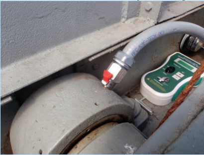
ADB Sensor Installed on Conveyor Bearing
